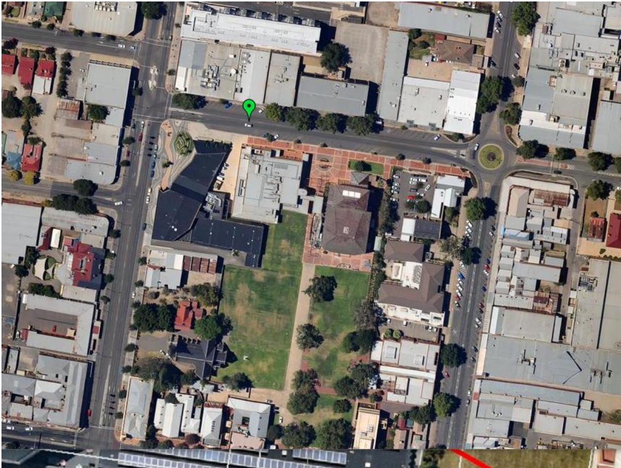
Figure 6: Aerial photograph showing that the southern wing of the AEC was already demolished in 2010, by NearMap
